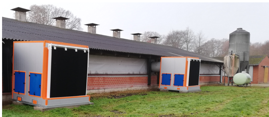
Figure 1: Two filter boxes for air supply installed at one side of a naturally ventilated turkey barn. The curtains remained closed during forced ventilation.
